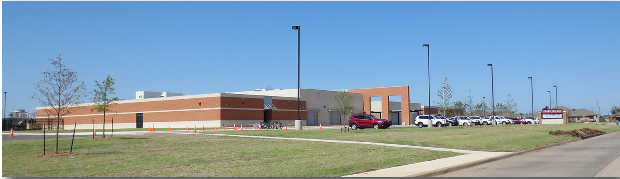
A completely new Plaza Towers Elementary School opened for classes in September 2014.
