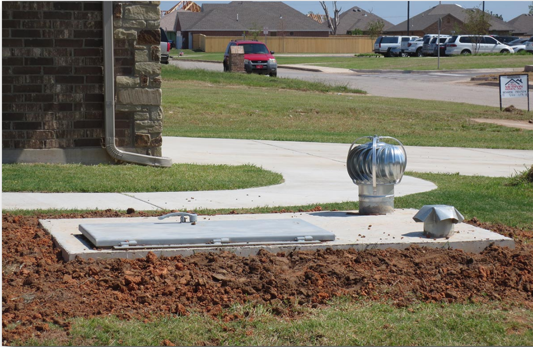
A close-up of an underground storm shelter in the front yard of a new home. Plaza Elementary is directly across the street.
