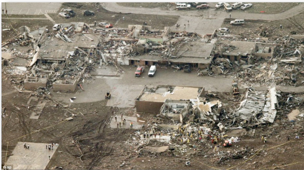
Plaza Towers Elementary School, pictured the day after the tornado struck in May 2013.
