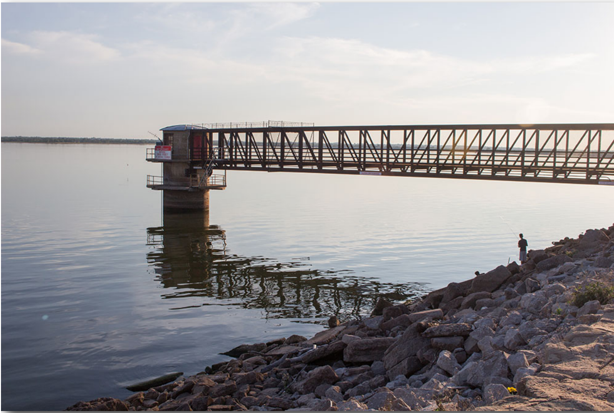
Lake Hefner is a man-made lake that supplies water for Oklahoma City's municipal water system. Pictured above is the intake tower for the water treatment plant located across the street.
